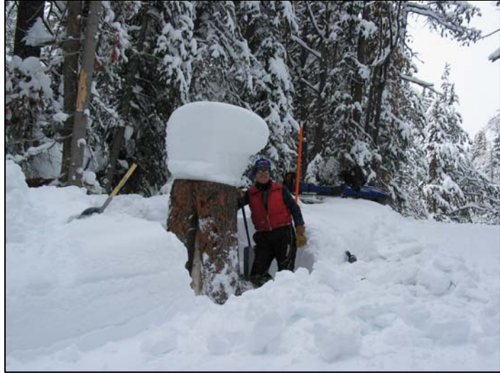
Photo 3.7 It is easier to remove stumps, brush, and debris before snowfall accumulates.
